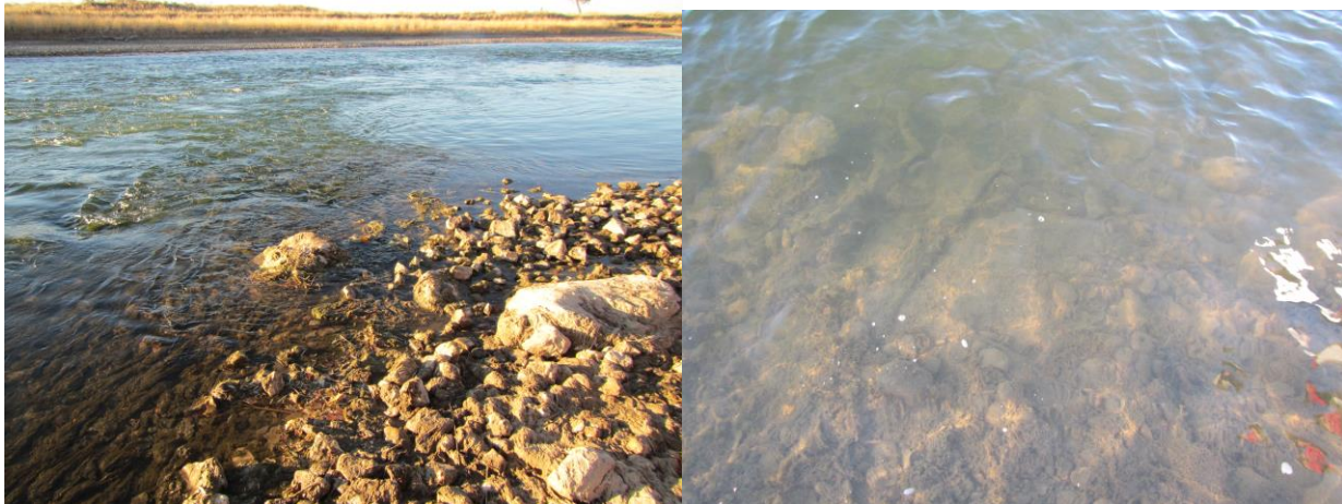
Figure A.3.2. Site 1 - Morad Park, standing on right bank, looking across the channel at Rock vane 1 (left). The header boulders are visible above base flow in the foreground (left). Boulders underwater at the same level of the surrounding substrate further into the channel (right).
