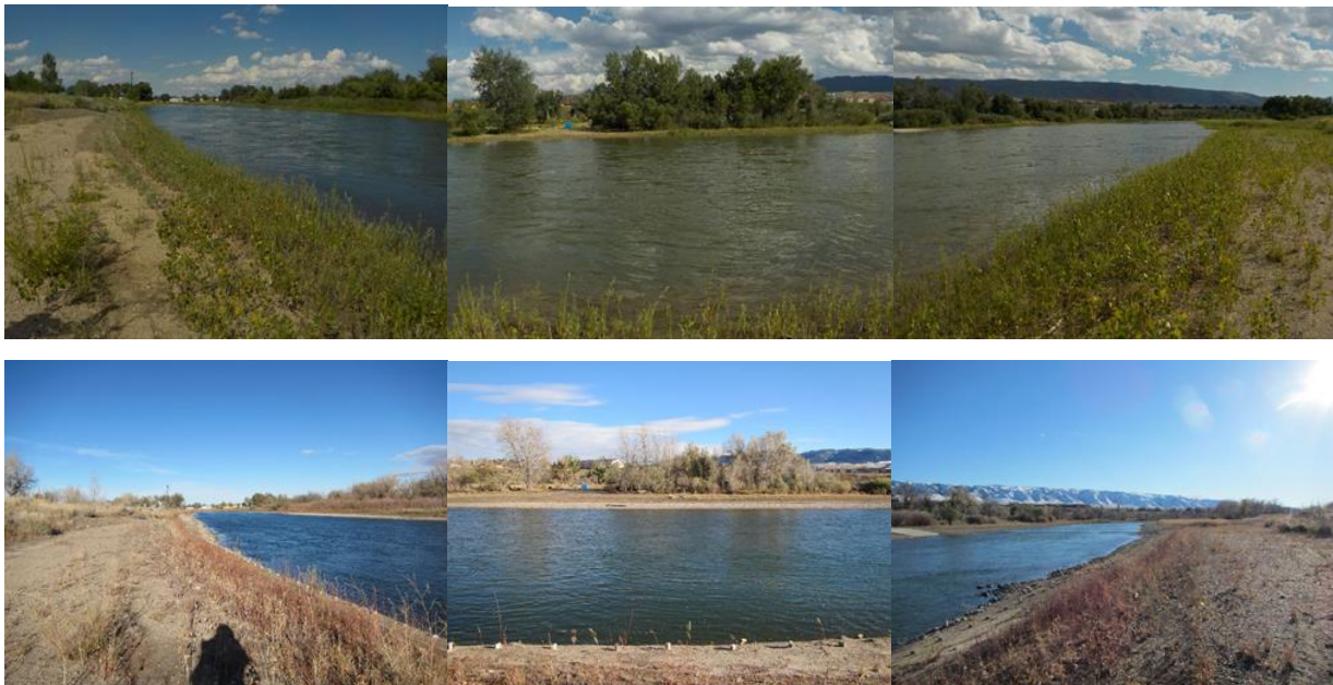
Figure A.2.7. Views from photo point MP-6 looking downstream (left), across (middle), and upstream (right). Many cottonwoods and willows are established and doing well both upstream and downstream. However, the top of these banks are still mostly bare. The upstream image shows the constructed riffle vanes, which continue to function to control the grade and direct flow to the center of the channel.
