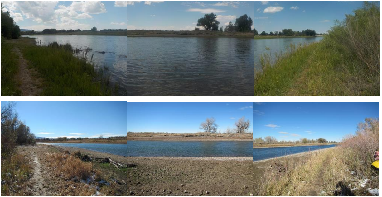
Figure A.2.5. Views from photo point MP-4 looking upstream (left), across (middle), and downstream (right). Vandalism in 2016 also resulted in loss of most stakes along this bank. Most of the vegetation establishment has been herbaceous, although many young willows have established downstream.
